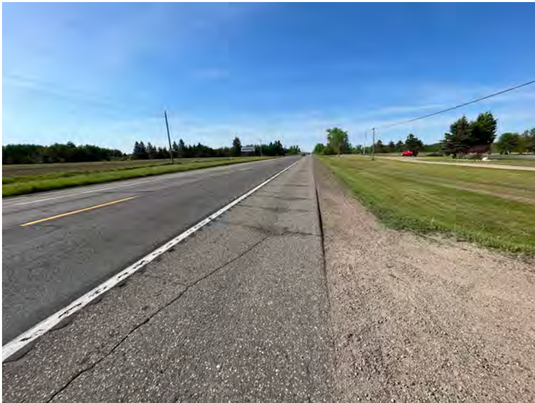
Looking south down US 71
