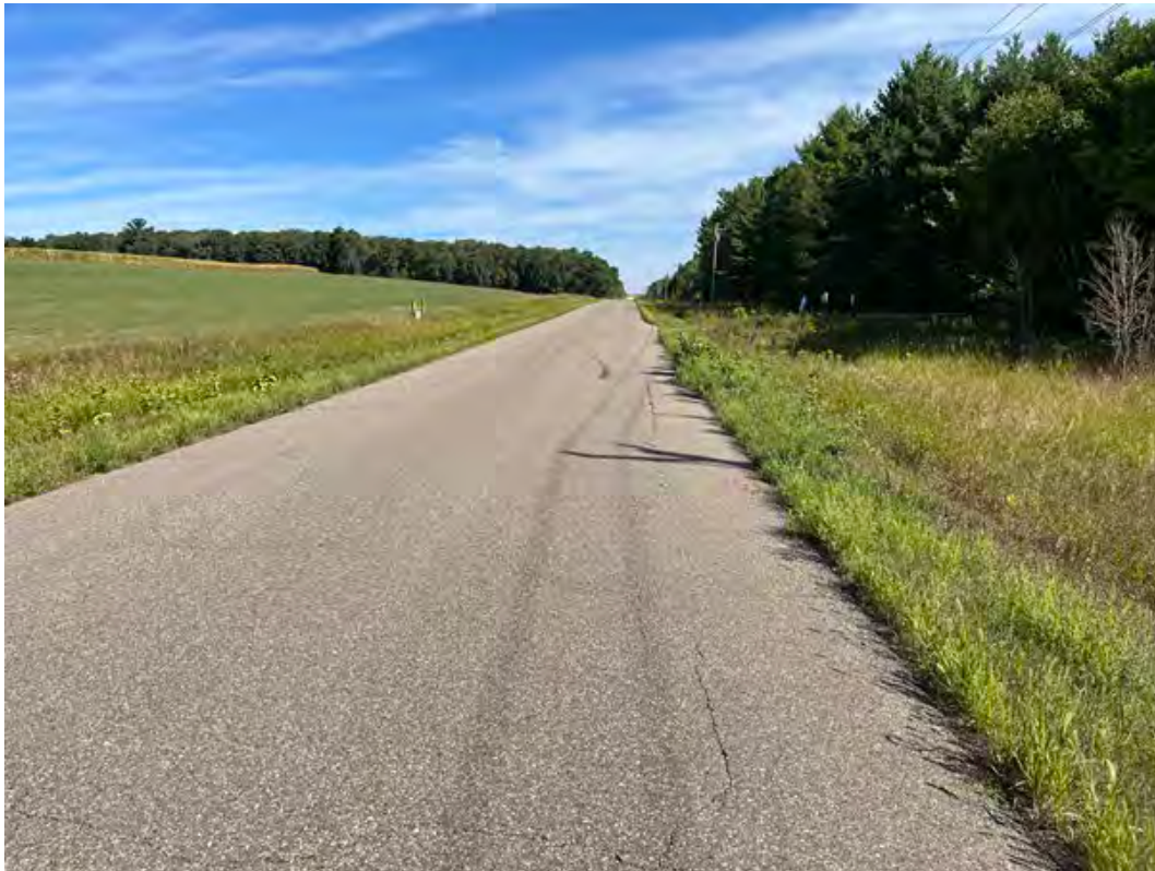
Looking north down 281 st Ave
