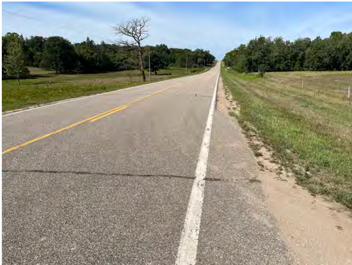
Looking west down 350 th Street
