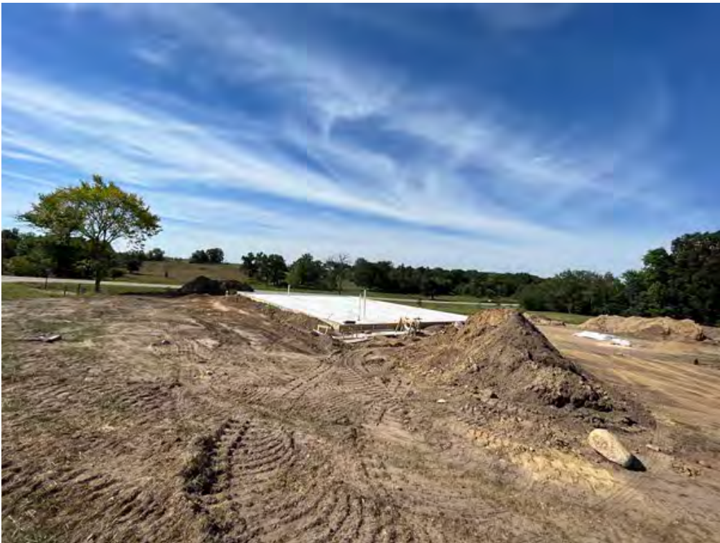
Proposed structure location for poly furniture construction
